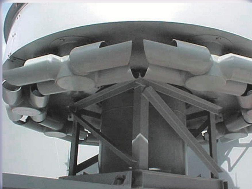
ENHANCED ENERGY DISSIPATING INLETS "Designs that allow sludge blankets to survive hurricanes."
